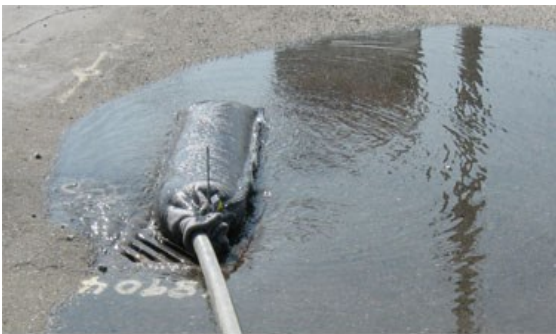
8" dia. x 5' long Filter Sock remove oil and suspended solids from water
