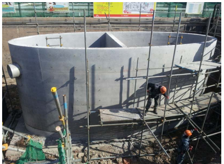
<Completed oval structure of AOS SEPARATOR only>
