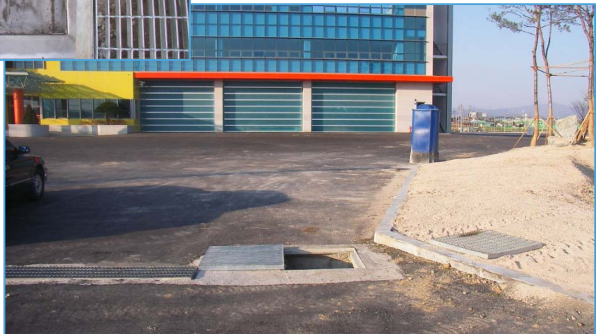
<collecting well type of non-point pollutants treatment equipment of construction site of Yeongcheon Fire Station>
