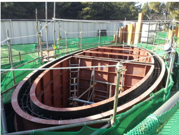
<Installations of oval steel form>
