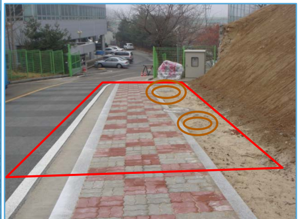
<After completion of construction work>
