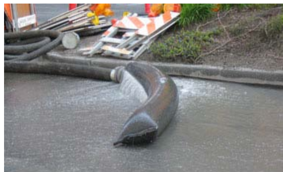
8" dia. x 10' long Filter Sock remove oil and suspended solids from water
