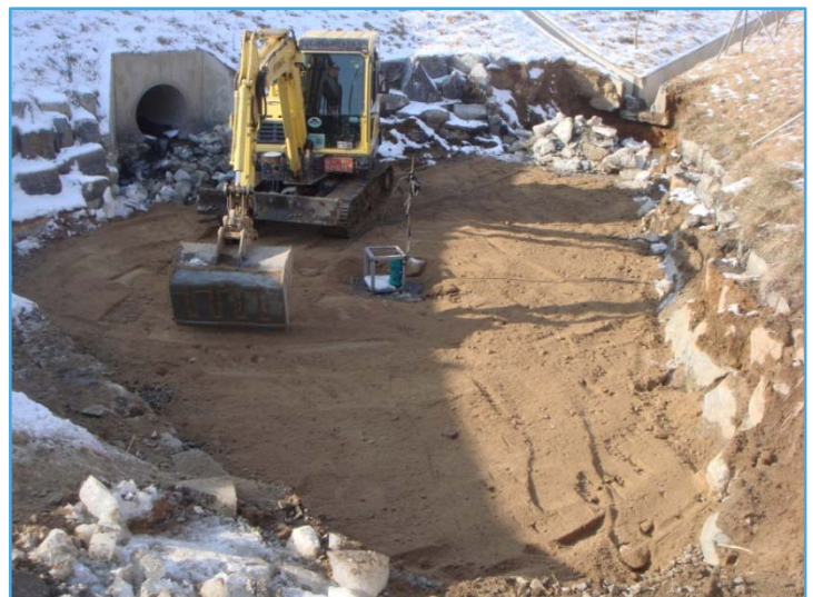
<Construction of vegetation soil zone>
