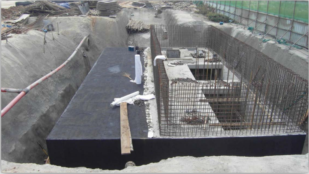
<Installation of AOS SEPARATOR structure>
