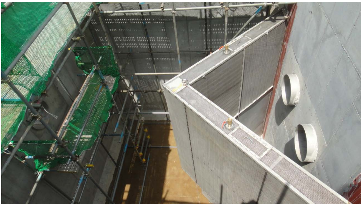
Construction of AOS SEPARATOR (SK Energy)
