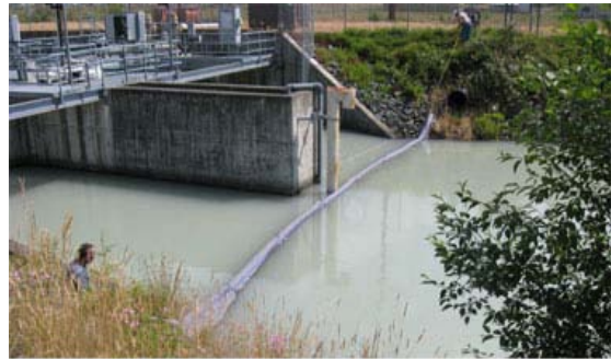
Filter Booms connected units spanning river
