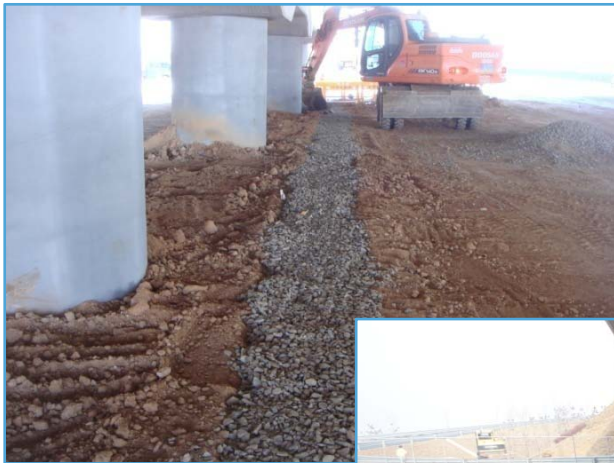
<collecting well type of non-point pollutants treatment equipment of construction site of Yeongcheon Fire Station>
