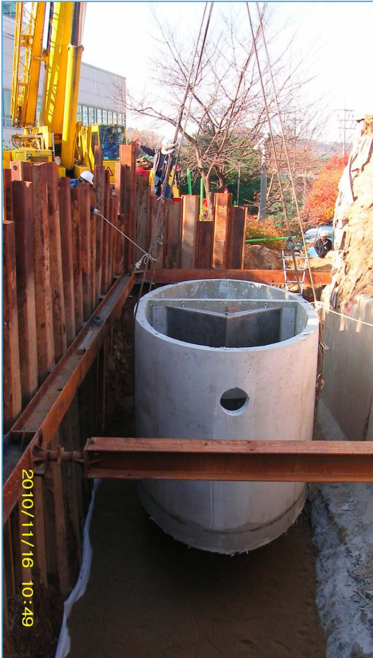
<Installation of body of treatment facility>
