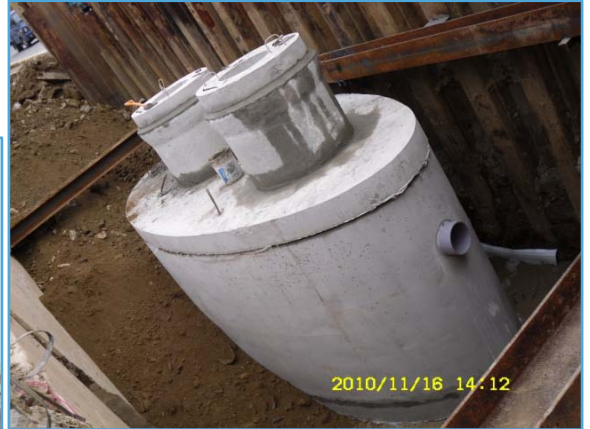
<installation and backfill of inspection opening>
