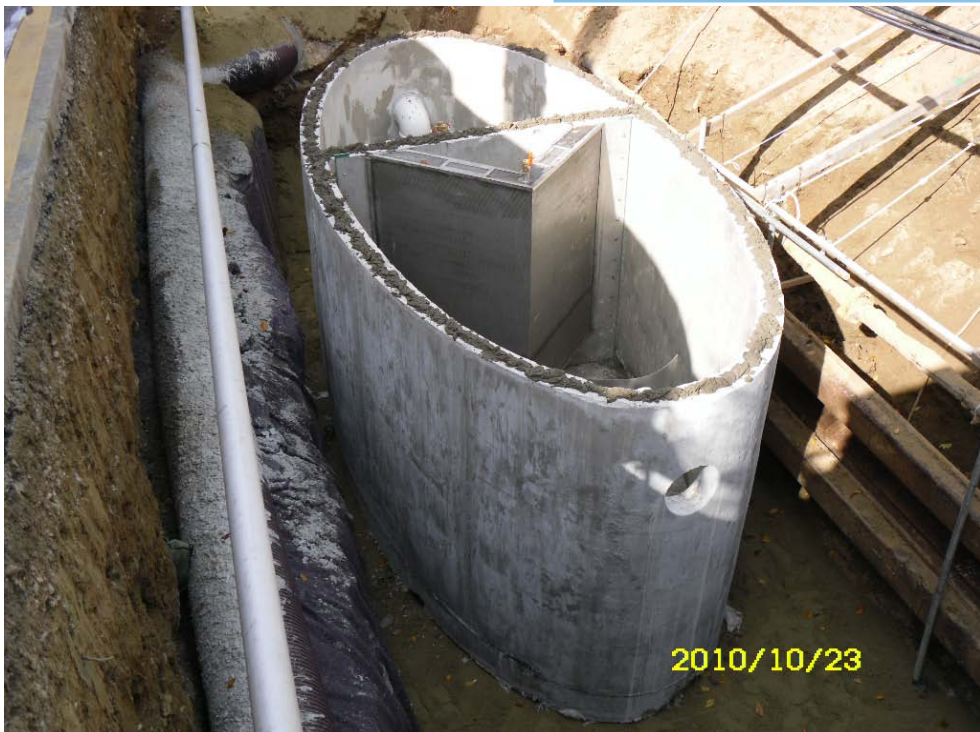
Construction of AOS SEPARATOR
