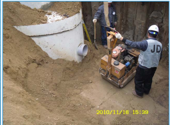
<compaction of embankment>
