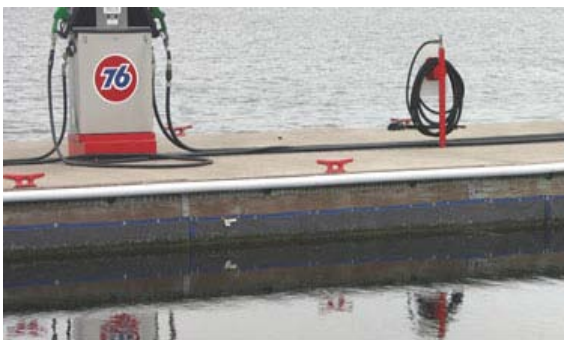
Boom and Dock Curtain continuous collection of oil & sheen at fuel dock
