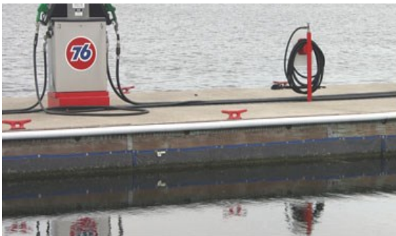
Boom and Dock Curtain continuous collection of oil & sheen at fuel dock
