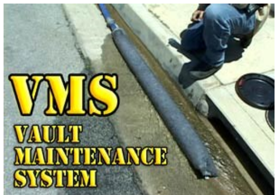
Shore Guard aka "Dumbo Surfer" connected units - 10" overlap - stainless steel clips
